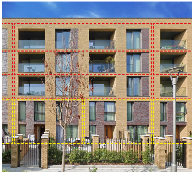
Figure 173 Modern residential block with front door maisonettes on the lower two floors and internally accessed apartments on the upper floors
